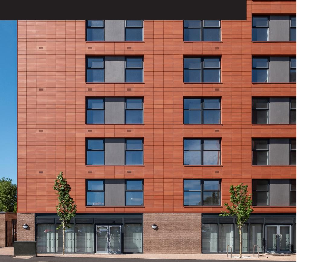
Taylor Maxwell worked with **Willmott Dixon** and **Longworth Building Service** to specify and supply Argeton terracotta cladding in Salmon Red and Ferro Grey to the £22.5m project. The terracotta rainscreen system was expertly installed by Longworth Building Service.
