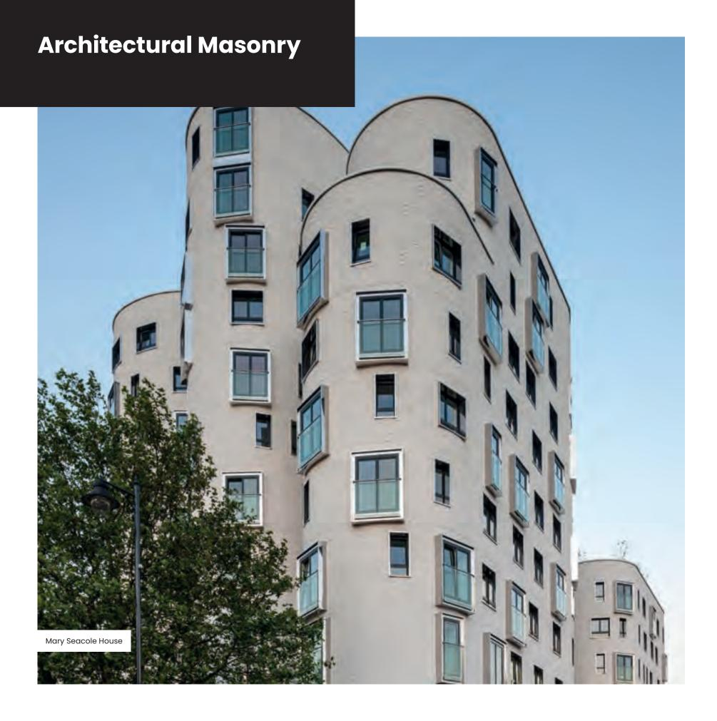
Architectural masonry provides a decorative facing concrete block with design quality and dimensional accuracy. It is a structural material which can be used as part of the internal or external leaf, providing a clean, maintenance-free solution.
