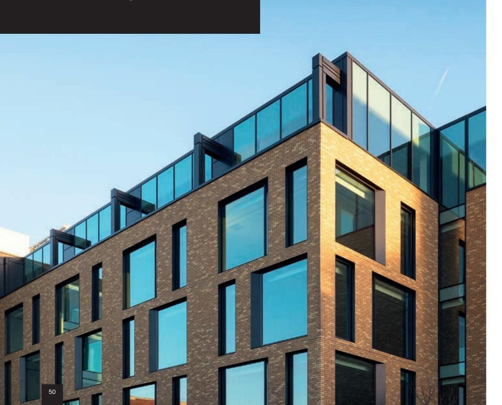
The tired 1980s office block facade of Belmont House was stripped back to the original concrete frame to facilitate the modernisation of the dated design and provide a fresh and efficient first class office building for the area, designed by architects TP Bennett for their client Aviva.
