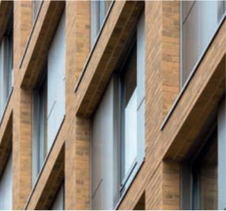
Mounted at an angle or as a soffit, CORIUM can achieve a dynamic finish. Mosaic and decorative patterns can add an extra dimension to any project. For further detail on installing CORIUM at an angle, please get in touch and we will put you in contact with the relevant specialist.
