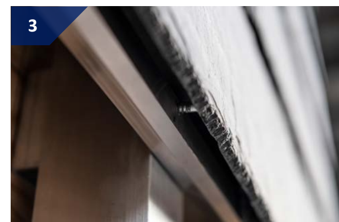
Cut the screws holding the broken slate with the saw
