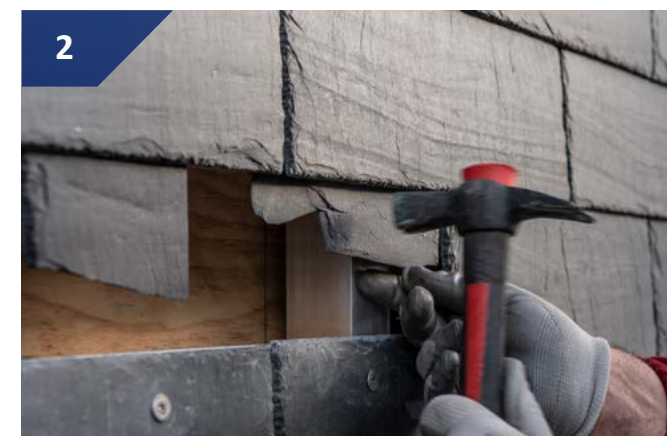
With a hammer, remove the broken pieces of the slate
