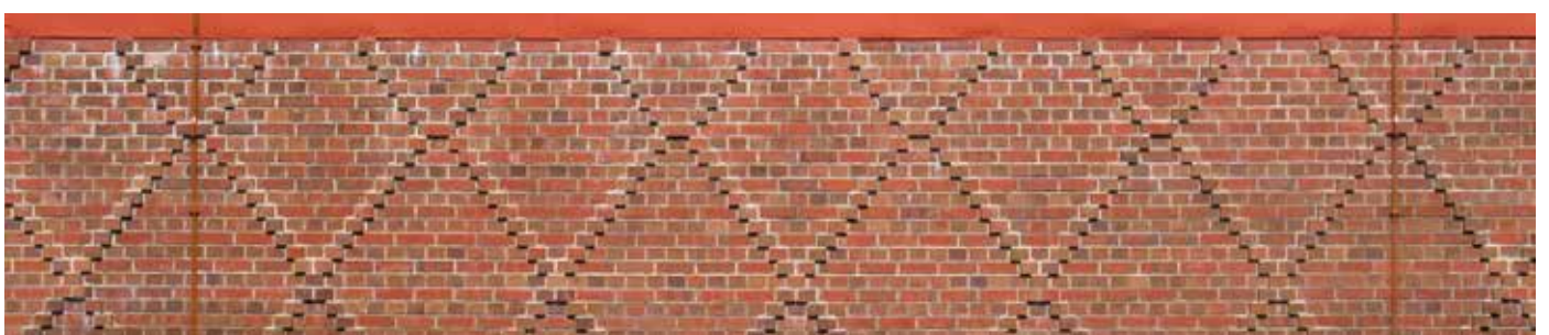
St Luke's Church, Blackburn - detail. Patrick Wilson Architects.
