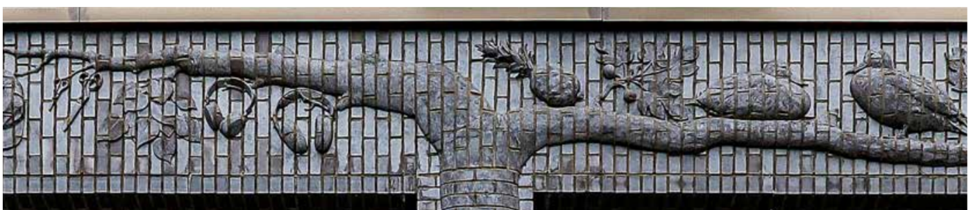
Peabody Burrige Gardens. Ibstock bespoke brick. Hawkins Brown Architects. - Detail of bespoke brick
