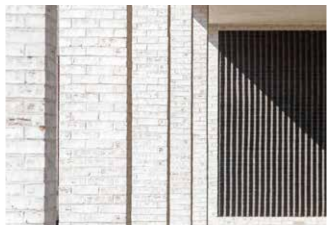
Travelodge, Rochester. White Brick and Mortar - Detail
