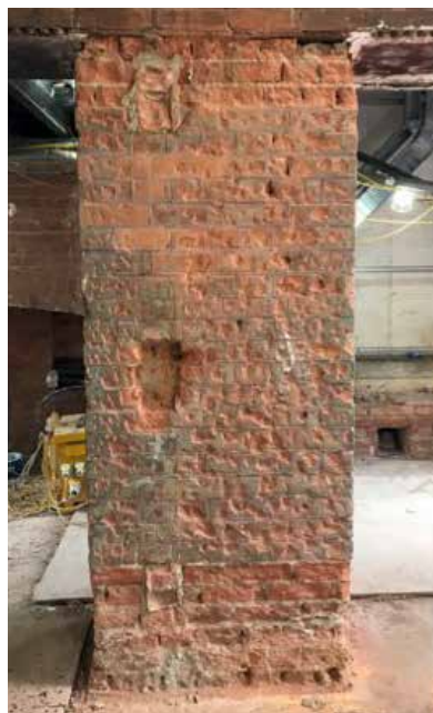
Leighton House Cafe Refurbishment Original bricks
