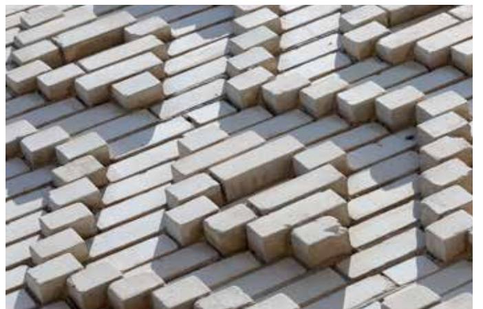
Example of Protruding 'Diamond' Pattern - Detail
