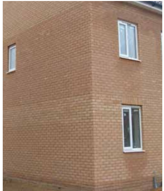
Poor Practice showing bands of unblended bricks
