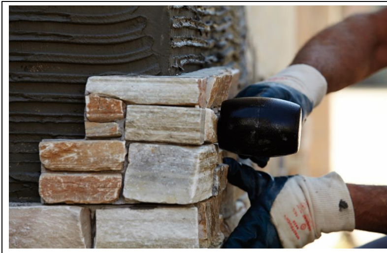
Figure 5 Stone panels bonded to the wall
