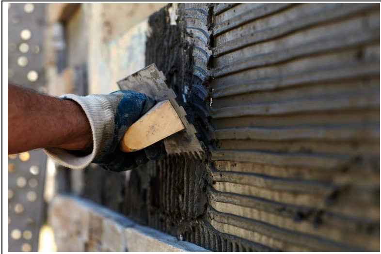
Figure 5 Stone panels bonded to the wall
