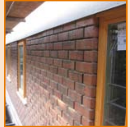
Windows fitted into existing spaces in Gebrik
